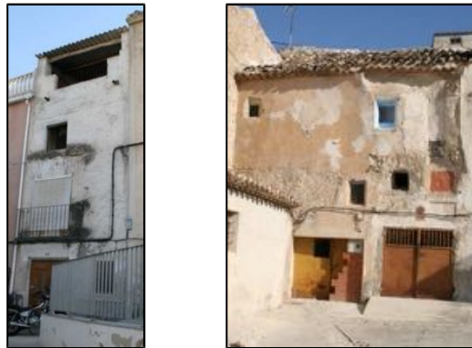
Figure 8. Images of buildings with no registered residents (own photo)
