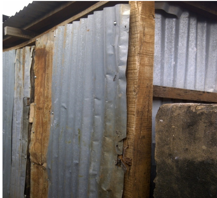
Figure 1: A typical latrine in the community Source: Authors' Field Work (2013)
